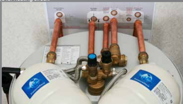
Top valve, expansion vessels and coil connections
