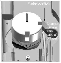
Using cylinder thermostat as high limit stat only - coil the grey temperature probe wire inside thermostat box and insert black probe into thermostat pocket of cylinder then turn dial on front to number 5
